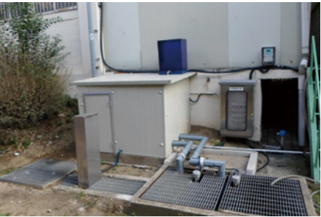
System that automatically closes the rain water sluice gate
